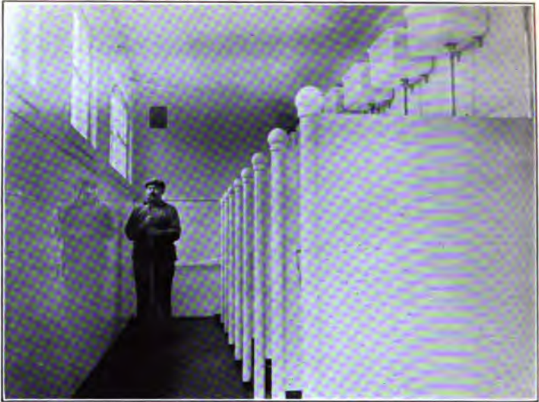
CLOSETS IN COMFORT BUILDING AT LUCY FURNACE
